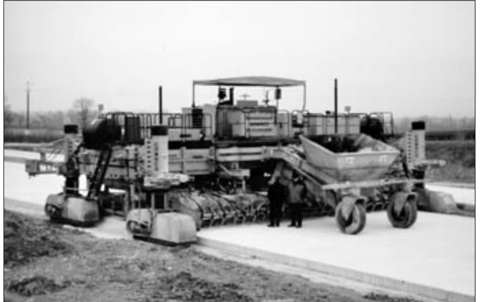
The Gomaco 4000 paving machine set at 10.75 m wide for this contract – stood down due to cold weather.
