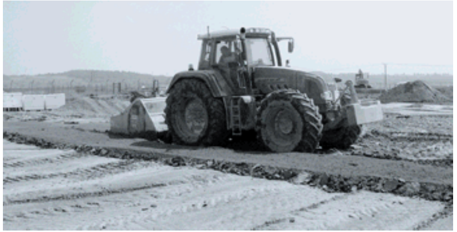
Incorporating PFA into the soil.
