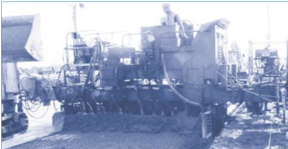
Slipform paving at the London City Airport
