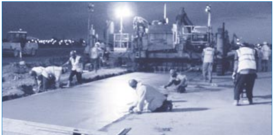
Overnight paving at London City Airport
