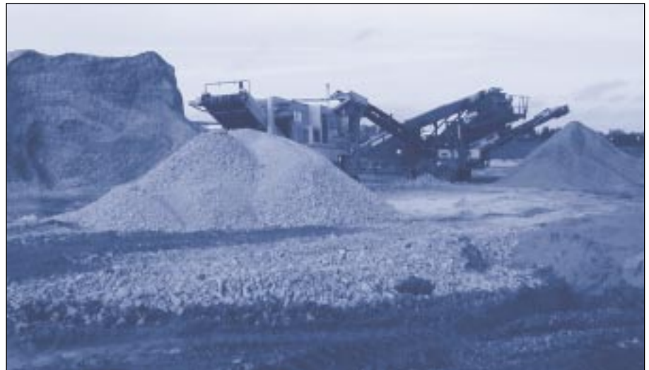
Re-processing the crushed concrete to below 40 mm
