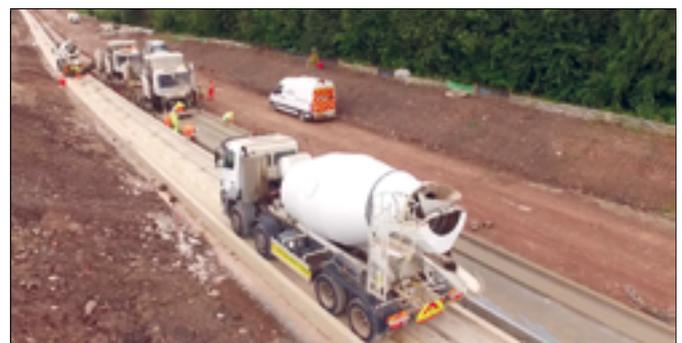
He continued: "The benefits of slipform are not just economic. The true achievement is the smoothness of the passengers' ride thanks to the lack of joints. Previous busways constructed from precast concrete blocks do not meet the exacting tolerances that have been achieved on this project because they feature frequent transverse joints and can, over time settle out-of-line. The slipform and grinding combination ensures the greater tolerances necessary for a smooth train-like ride."
