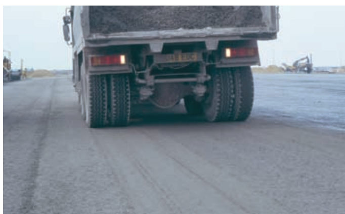
Figure 7: Mixture M10 showing improvement under tyred traffic after vibrating roller compaction
