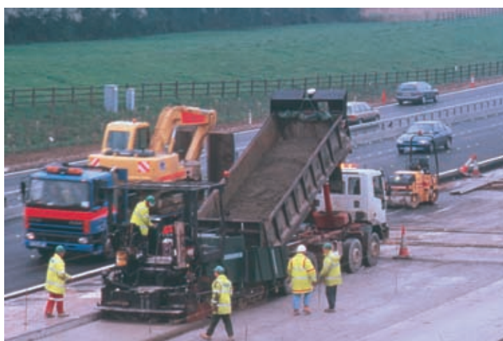
Figure 2: M25 Reconstruction, Clacket Lane, 2001 – fresh FSBM being overlaid by CBM
