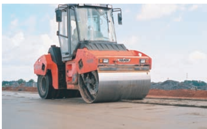
Figure 5: Mixture M5 showing shearing under roller
