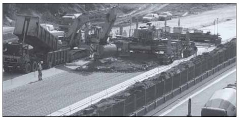
CRCP with low noise running surface used for rehabilitation of the Antwerp Ring Road
