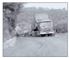
Reconstruction of the A52 in Staffordshire, where planings used as the aggregate were relaid after stabilisation off-site with lime and PFA.
