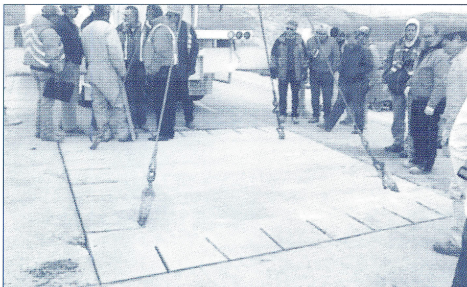
The new slab has been lowered into place – note slots precast into it, which will be matched by similar slots cut into the existing highway
