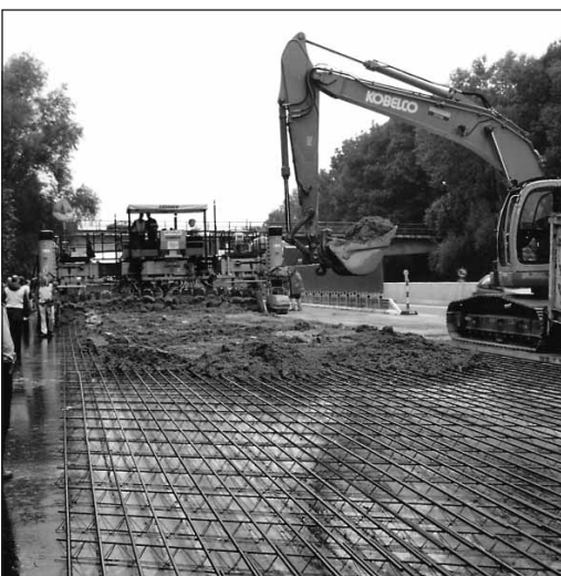
Concrete being placed by bucket in front of the paver.
