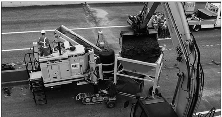
Slipforming the Dutch step barrier.
