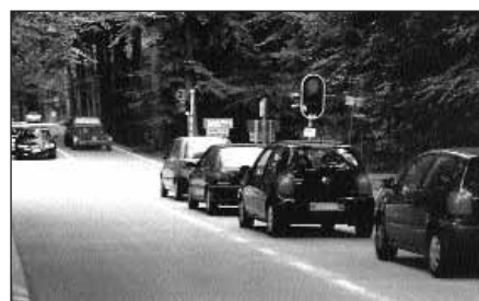
Lorraine Avenue – new overlay on Belgium's oldest concrete road, in use since 1925.
