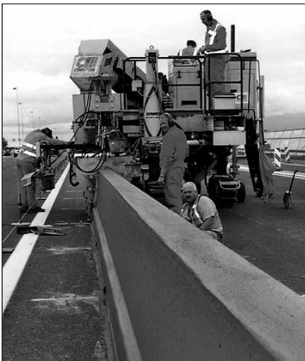
Slipforming a step barrier in the Netherlands.
