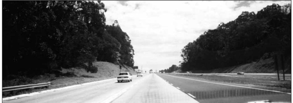
Low maintenance truck lanes keep the traffic flowing up the steep incline inland from Durban.
