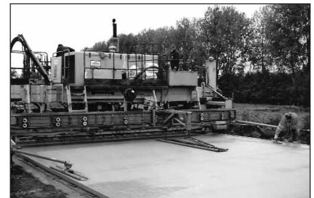
Following up with hand finishing.
