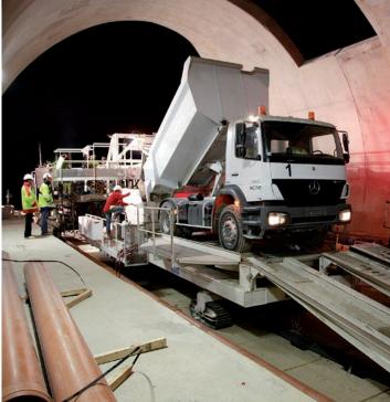
first of the side profiles to be slipformed was a slotted drain with a 250 millimeter (9.8 in) diameter. The profile is designed to drain away any dangerous liquids that could potentially spill from the goods transport trains. The slotted drain was slipformed the length of one tunnel. Then the Commander III would be moved to the adjoining tunnel and slipform the drain back in the opposite direction.
