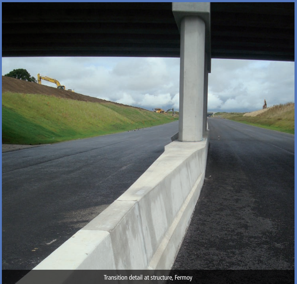
Barrier on concrete base foundation on the N6
