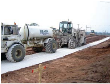
Mixing the water into the cement-treated capping layer
