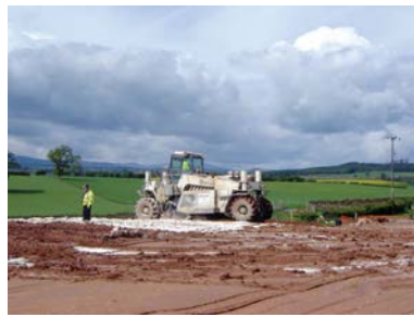
The Wirtgen mixing lime into a treated layer
