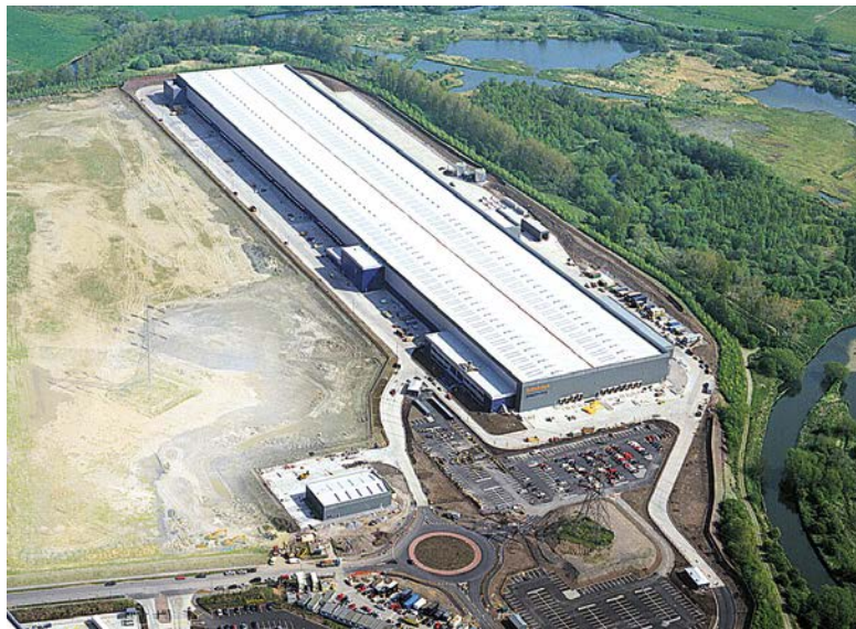
This large distribution centre was successfully completed to a tight programme (The area to the left is another plot yet to be treated)
