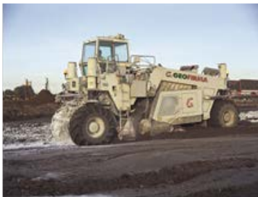
Incorporating the cement into the pulverised fuel ash
