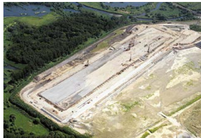
Arial view of the site showing stabilisation in progress
