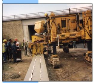
The pipe diameter will normally be 150mm or 300mm, but will need to be designed according to the run-off area, the outfall locations and the pipe gradient and characteristics. Sub-clause 517.20 requires that sections of the slot drain, not less than 500mm in length, are load tested. This imposes practical limitations on the size of the section which will normally be limited to a maximum diameter of 450mm.
